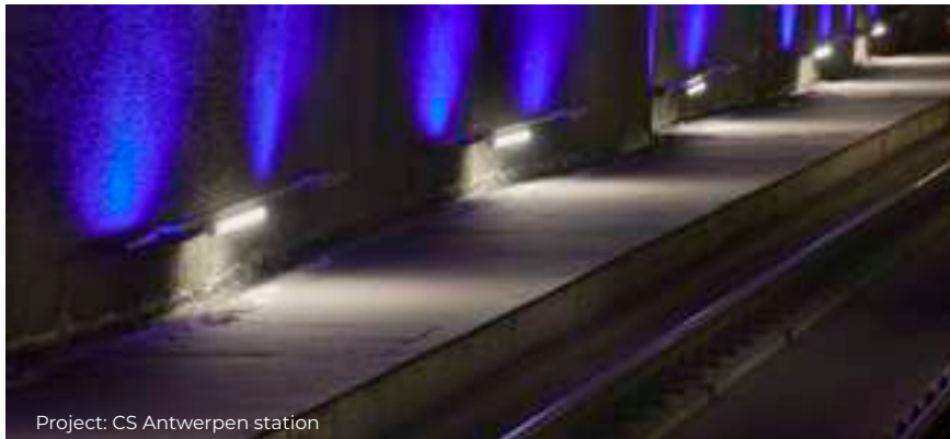
Project: CS Antwerpen station
